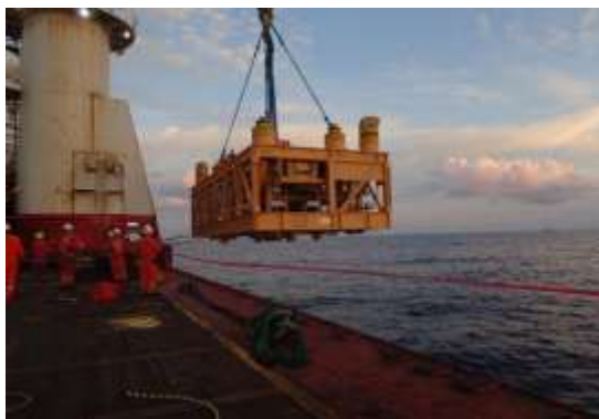
Manifold installation
