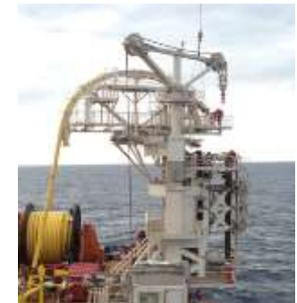
Flexible flowline installation
