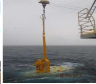
Transfer PLEM to lay tower
