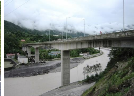
蔡家沟大桥 (Caijiagou Bridge)
