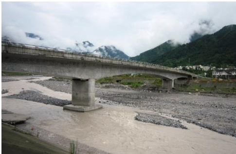
清平场镇大桥 (Qingping Town Bridge)
