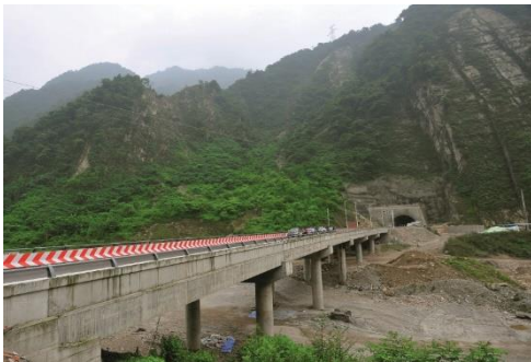
楠木沟大桥及金鱼隧道向清平出口 (NanMuGou bridge/ JinYu tunnel / Qingping exit)
