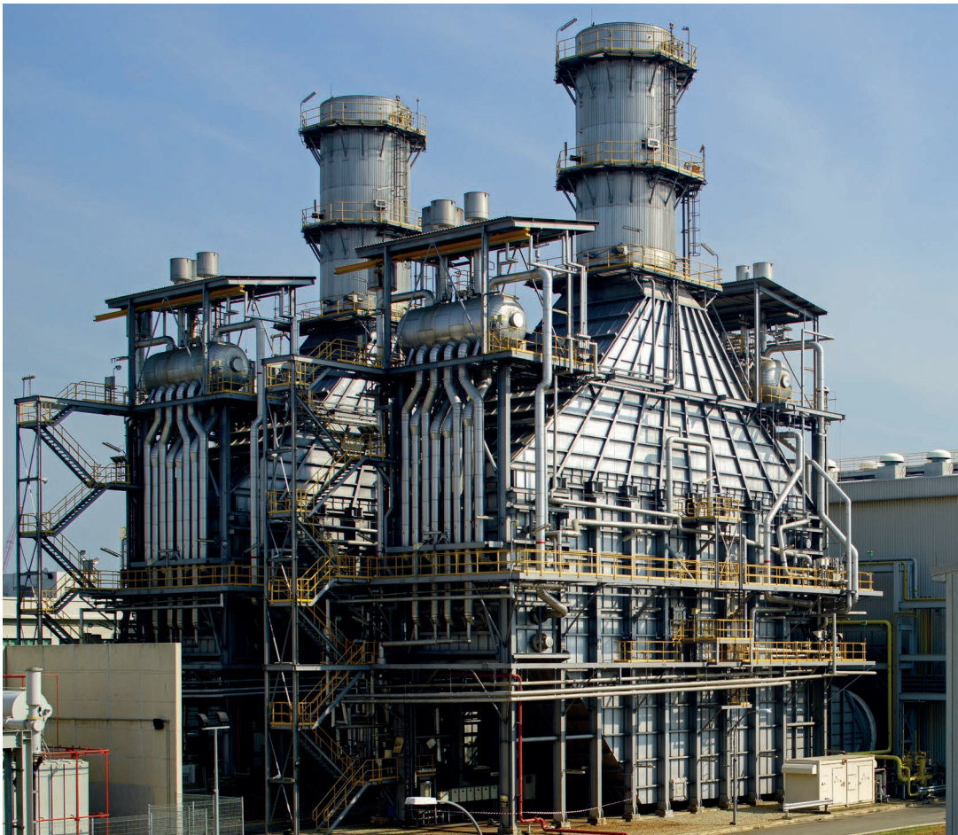
01 SingSpring Desalination Plant has been operating for more than ten years since commercial operations started in December 2005.
