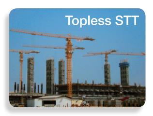
First introduced in 1999, the Topless STT's design features a streamlined jib design and no tower head, which minimises space to allow jib overflight of adjourning towercranes in a worksite. This makes the Topless STT towercranes particularly suitable for worksites with space constraints. The Topless STT towercranes are also designed to erect and dismantle quickly to save time which results in cost savings.
