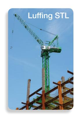
First sold in 2004, the Luffing STL towercranes offer a small slewing working radius due to a variable jib angle. This feature makes the Luffing STL towercranes particularly suitable for use in worksites that are surrounded by existing tall buildings or where jibs are not allowed to sail over existing buildings.
