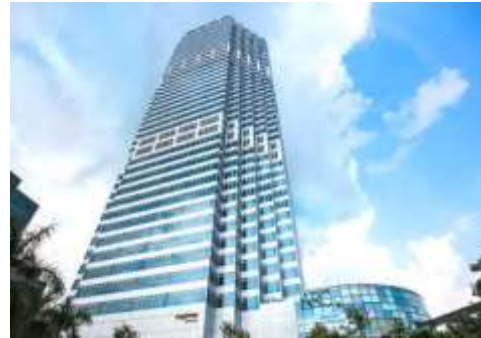
PSA Building S$740.8 million 3
