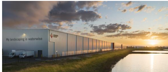
Leading position in industrial & logistics
