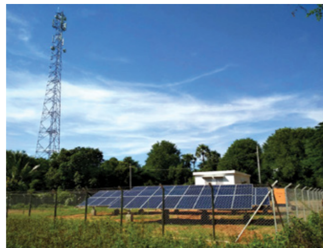
Yoma Micro Power supplying electricity to telecommunications towers.
