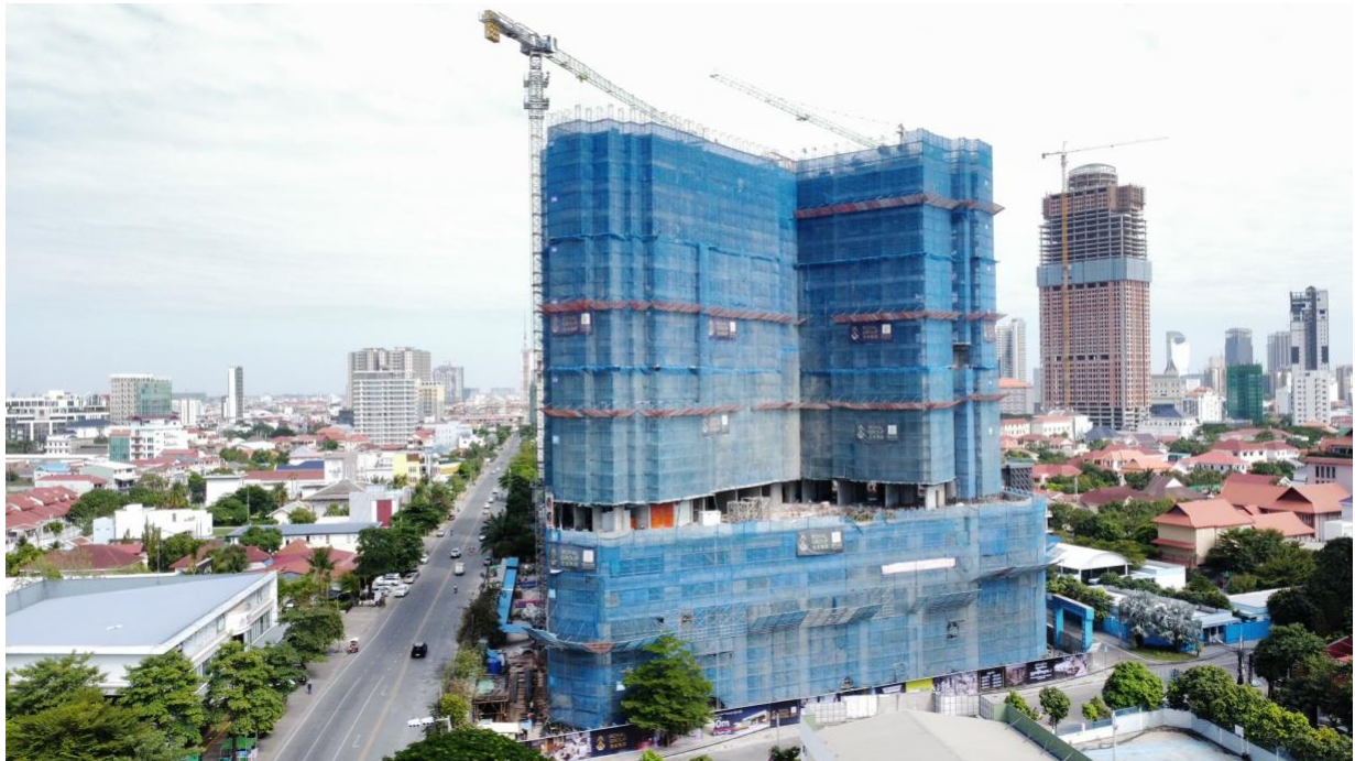
(Main Construction Site for Royal Platinum mixed-use project)
