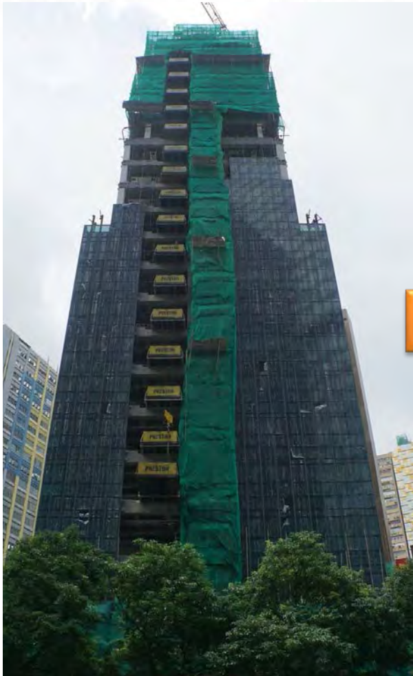
Existing site undergoing construction
