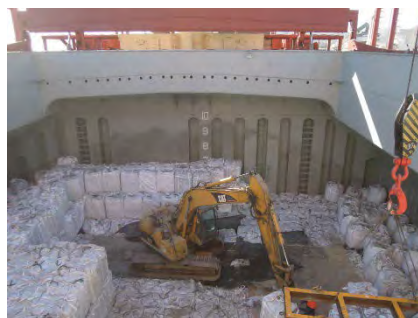
Loading bagged cement
