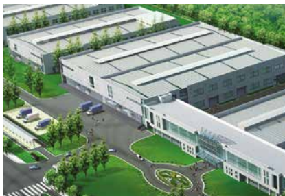
YHI ADVANTI MANUFACTURING (SUZHOU) CO., LTD
