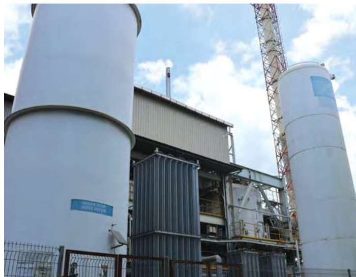
● Liquid oxygen tanks
