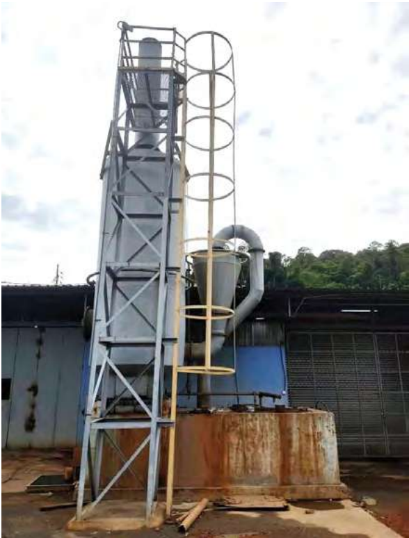
● Dust control system - Wet Scrubber
