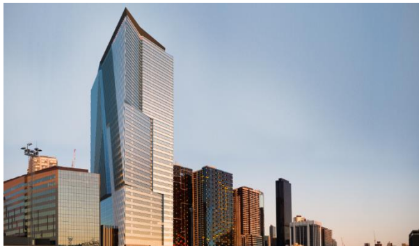
Topped out 311 Spencer Street in Melbourne
