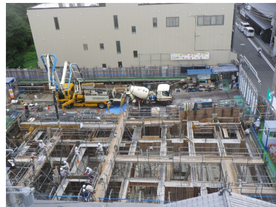
Existing site undergoing construction
