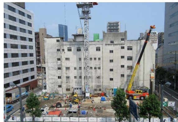
Existing site undergoing construction
