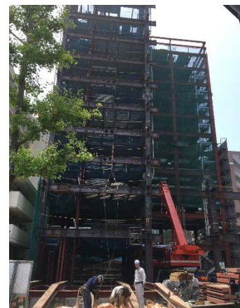
Existing site undergoing construction
