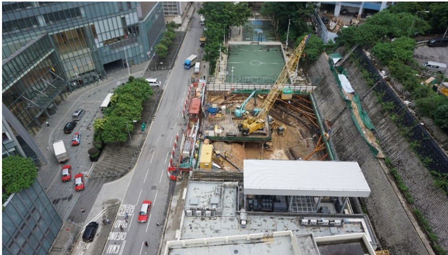
Existing site undergoing construction
