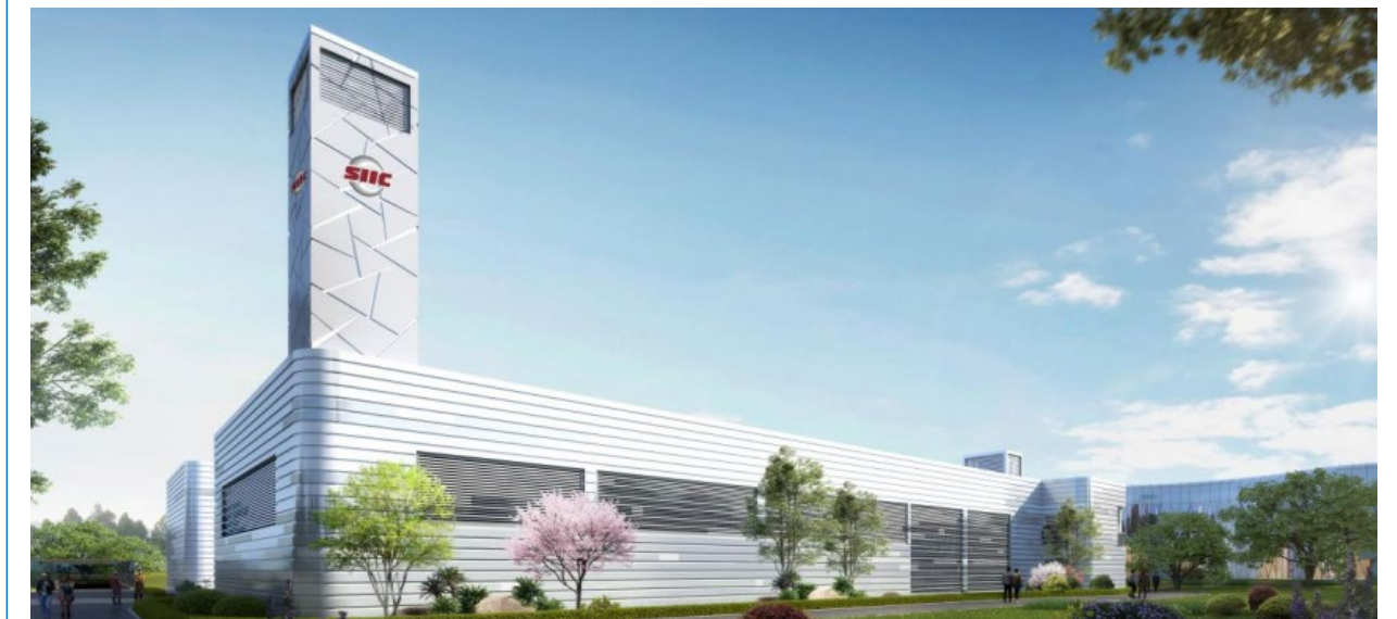
The Xicen Innovation Center Water Purification Plant
