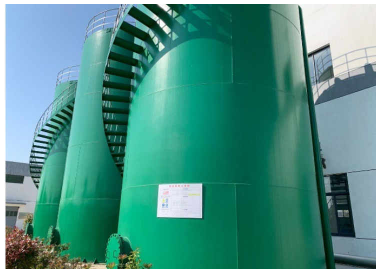
Taixing Huangqiao Industrial Park Water Treatment Plant water tank
