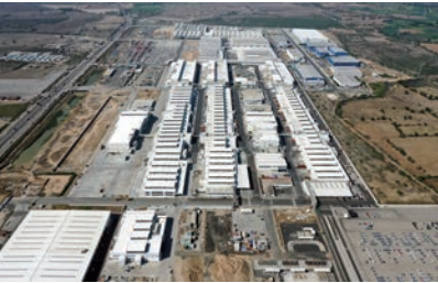
33 SUZUKI MOTOR GUJARAT PRIVATE LIMITED (Gujarat Plant)
