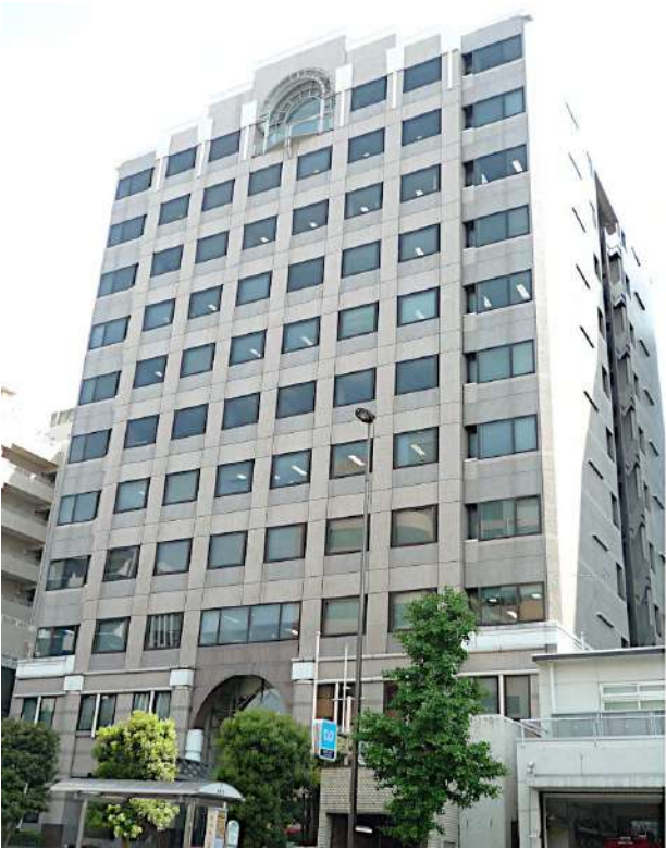
Narimasu Tosei Building
