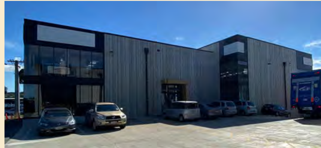
NEW ZEALAND WAREHOUSE
