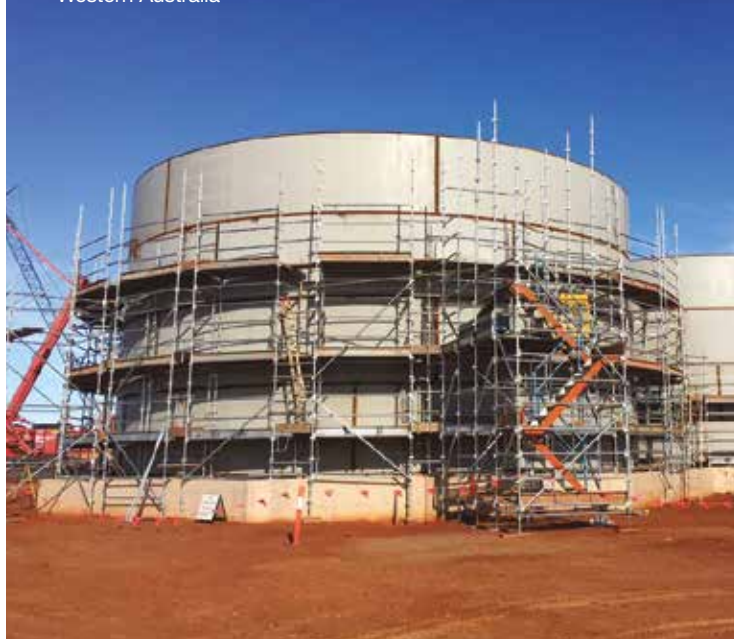
Gruyere Gold Project, Western Australia
