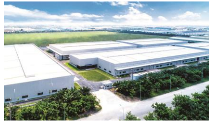
Phase 1 of Boustead Industrial Park (Vietnam)
