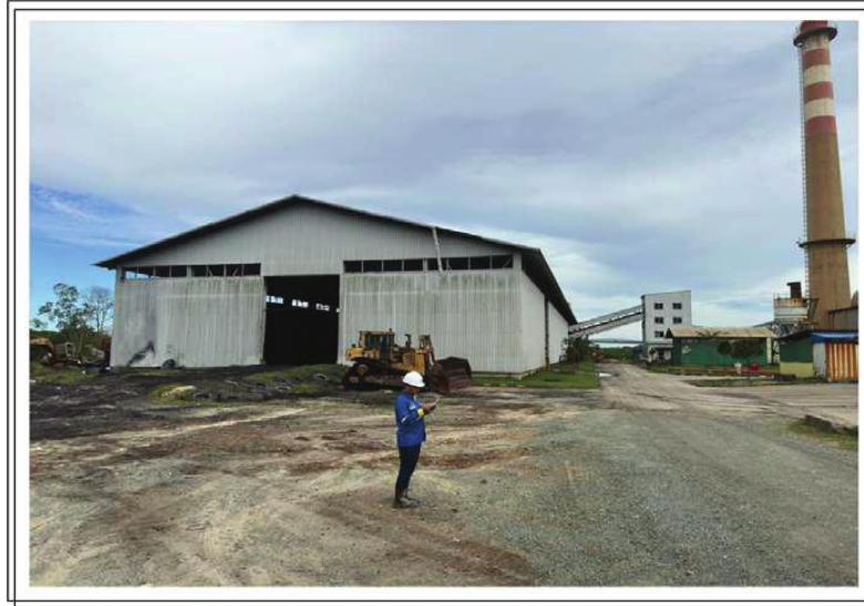
Coal Warehouse PT. Kariangau Power
