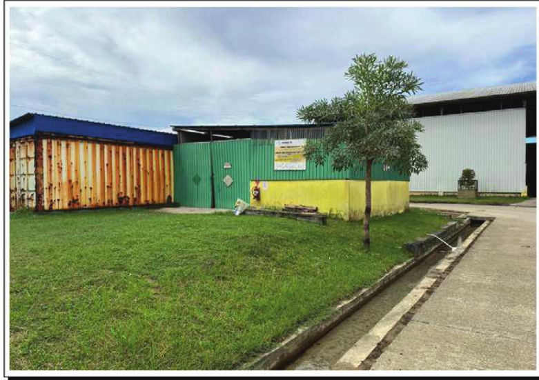
Toxic and Hazardous (B3) Waste Warehouse
