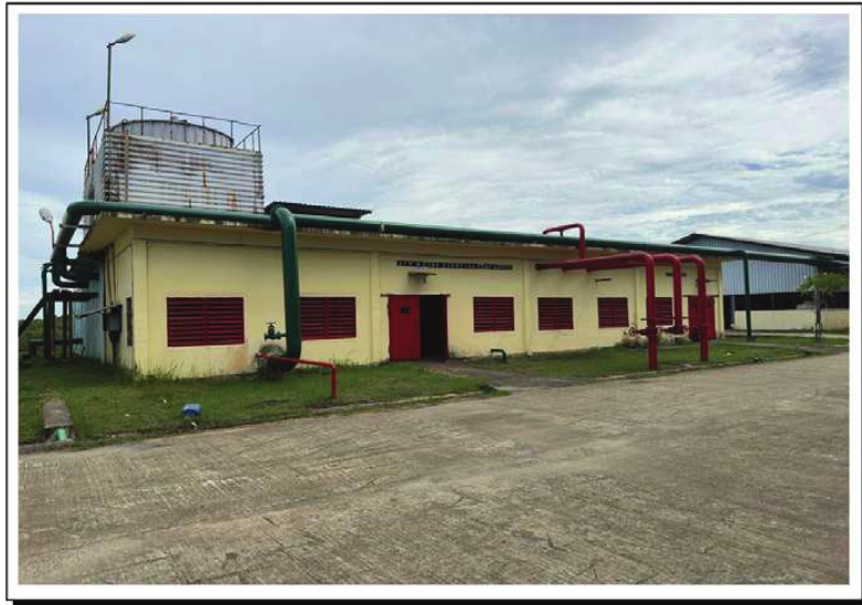
Fire Pump House
