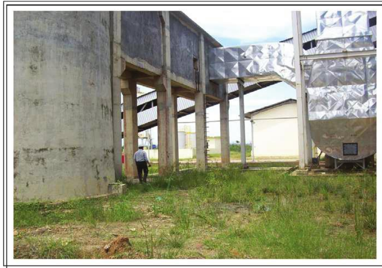
Flue Gas Duct Foundation
