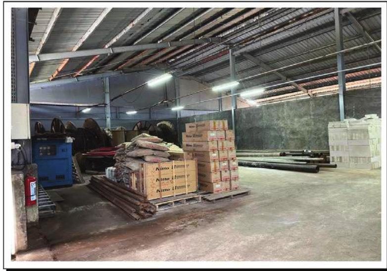
Warehouse I : Inside View
