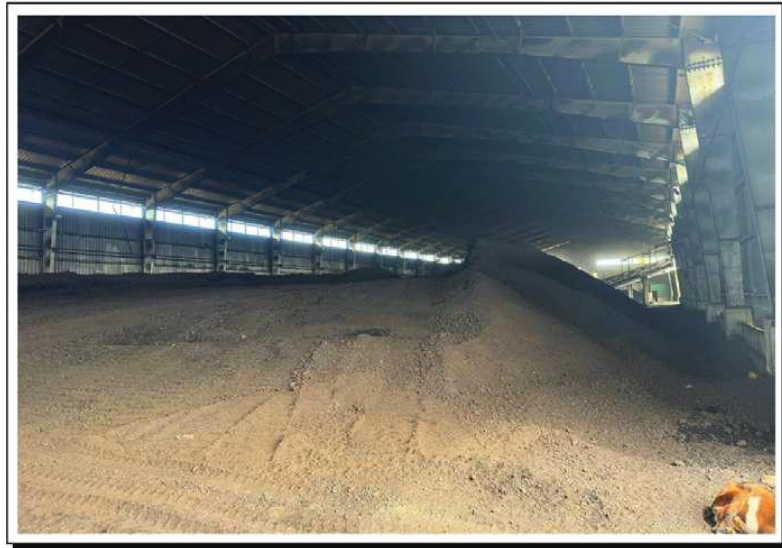
Coal Warehouse : Inside View
