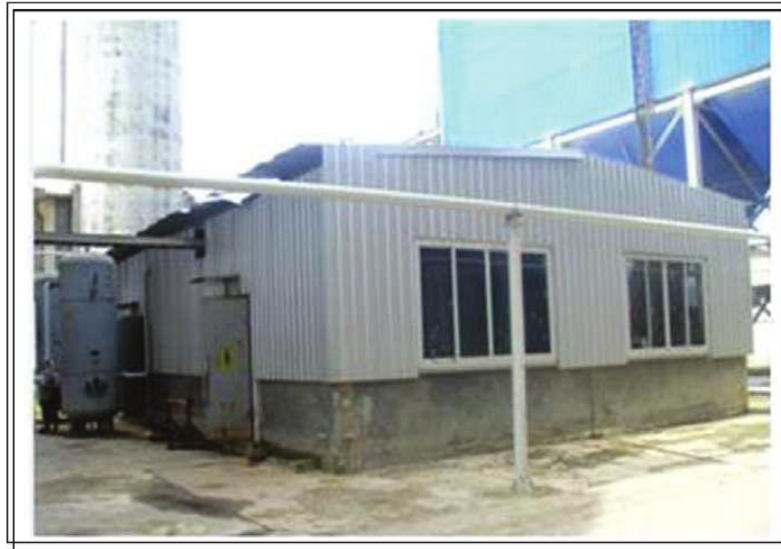
Air Compressor Room
