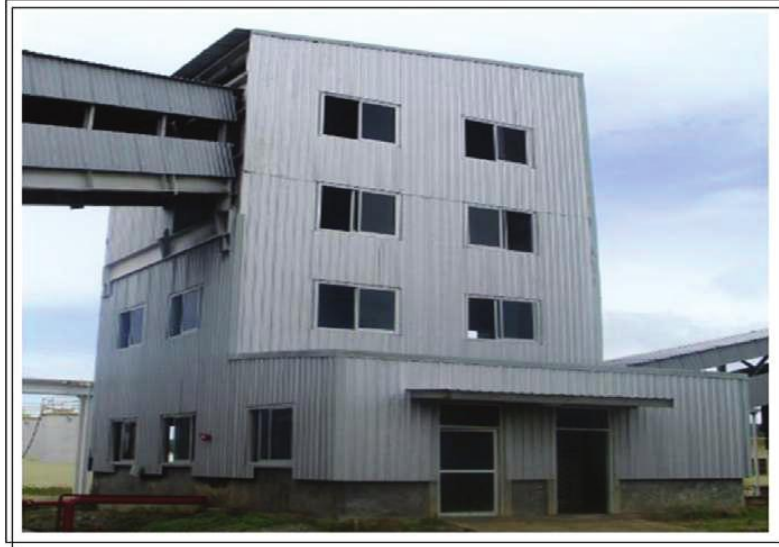
Coal Crusher Building
