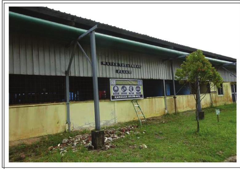
Water Treatment Building
