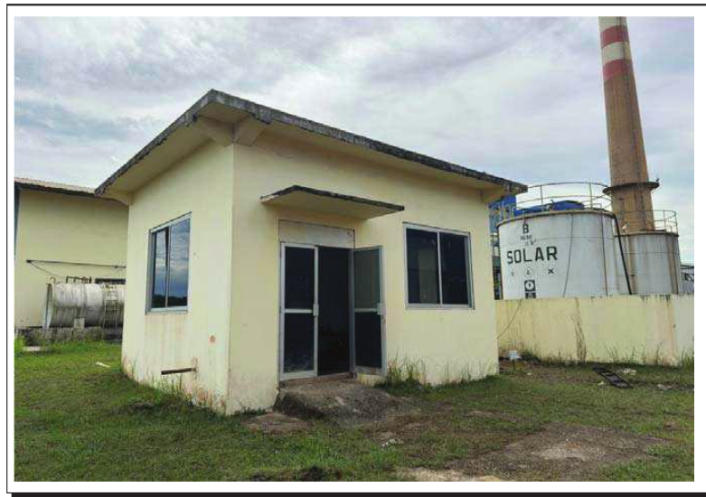
Solar Pump House
