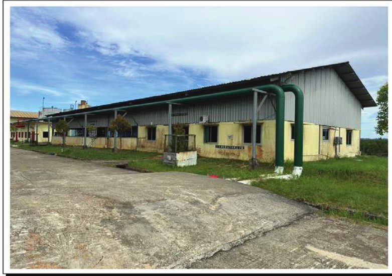
Laboratorium and WTP
