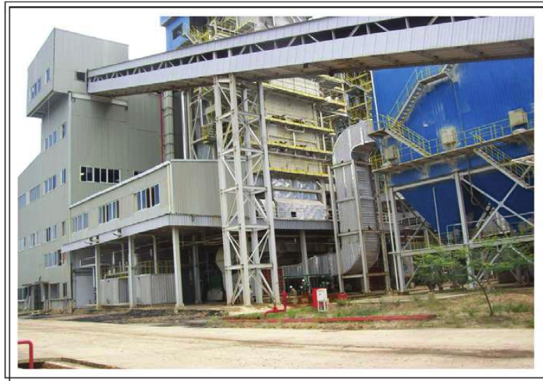
Coal Trestle (conveyor Galery)
