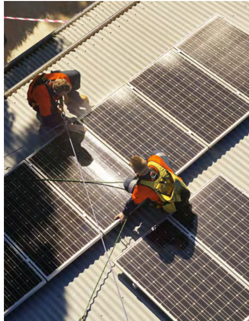
▲ We installed around 74 MW of solar on the roofs of Australian homes and businesses in FY2021.
