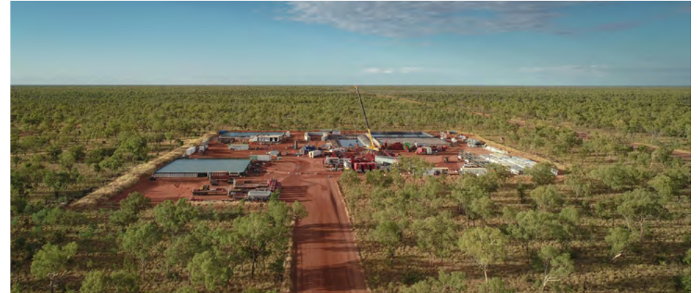
▲ Kyalla wellsite, Beetaloo Basin, Northern Territory.
