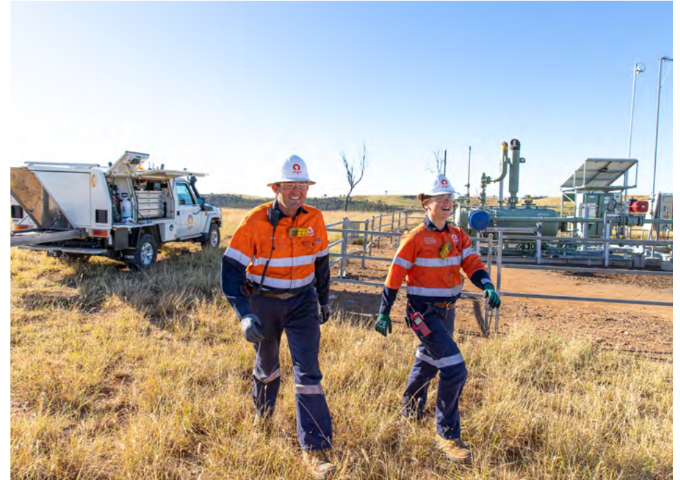
▲ Origin employees undertaking well maintenance in Spring Gully.
