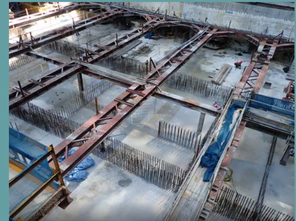
9000m 3 3-metre Thick Raft Foundation, CPF Tower (2018)
