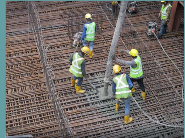
Low-Heat Concrete Pour of Raft Foundation, CPF Tower (2018)
