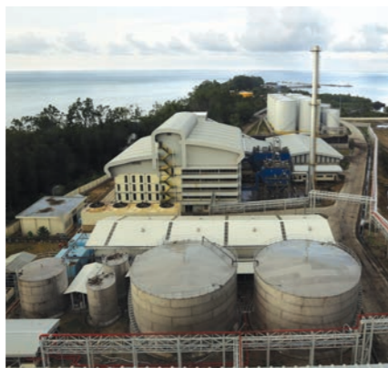
Palm Oil Refinery Indonesia
