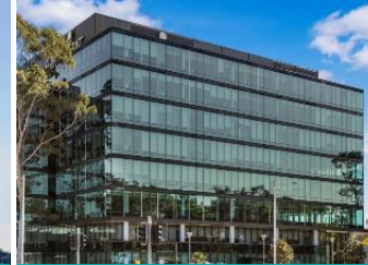
Dec 2020: Acquired Pinnacle Office Park in Sydney
