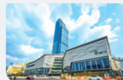
Spring City 66, Kunming—Hang Lung's first project in the Southwest region of Mainland China, has received LEED Gold pre-certification for Core and Shell Development issued by the US Green Building Council.
