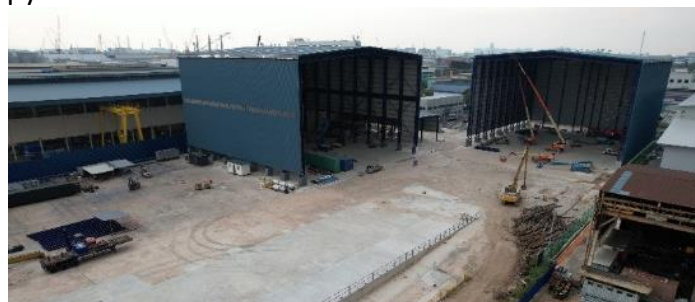
21 Tuas Road in early stage of works
