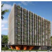
Crowne Plaza Changi Airport Extension (100% stake) 1
