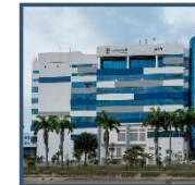
2 10 CHANGI SOUTH LANE
