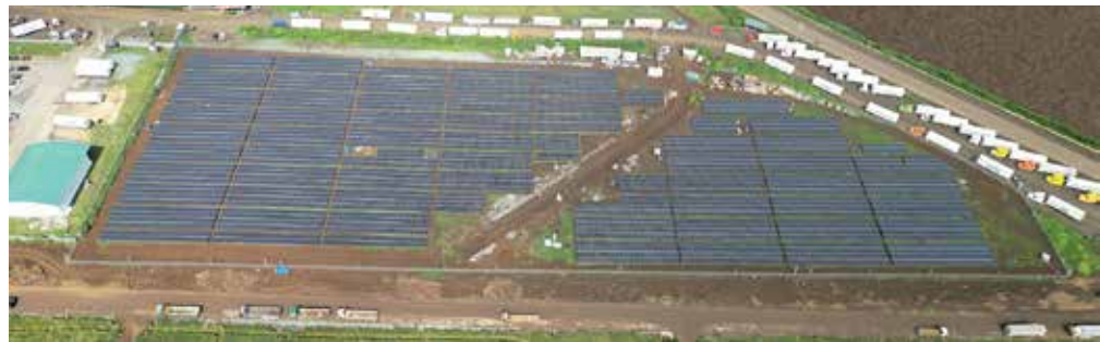
Solar energy facility near the Bukidnon manufacturing facility, Philippines
