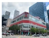
Cross Street Exchange
