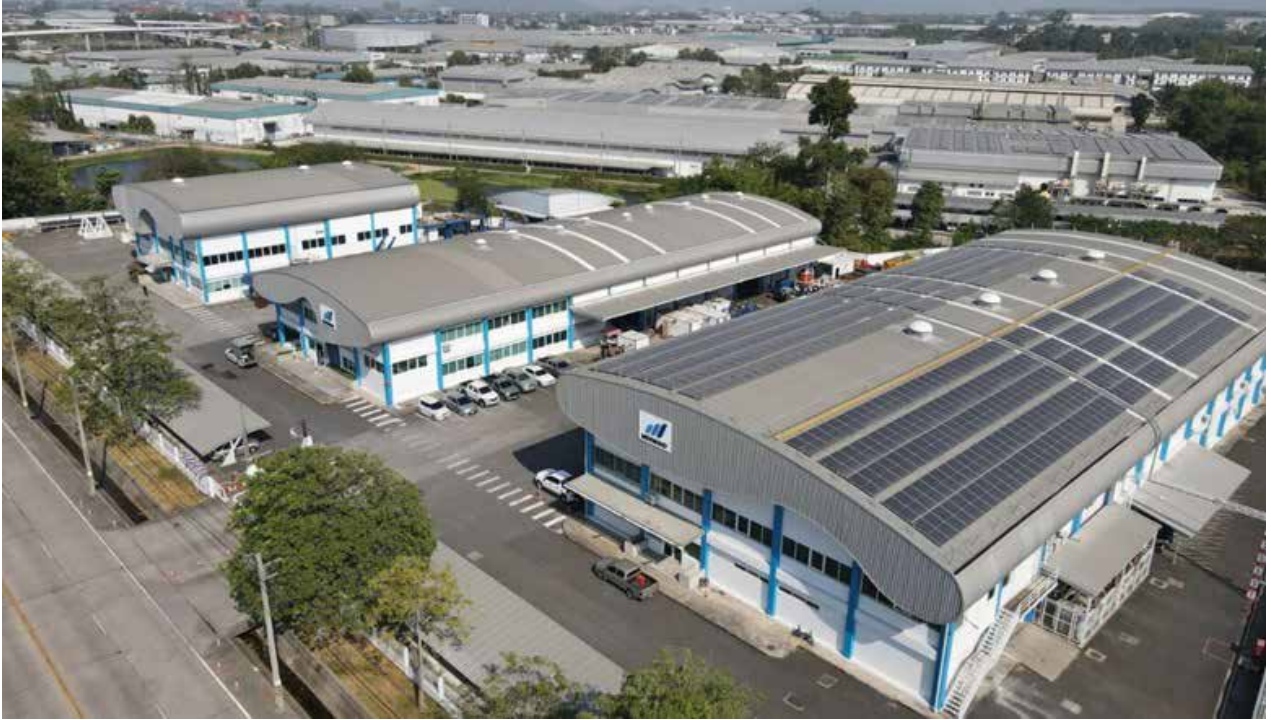
Figure 7 : Solar Panels Installed at Pinthong Office
