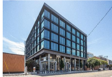
505 Brannan Street, San Francisco, US
