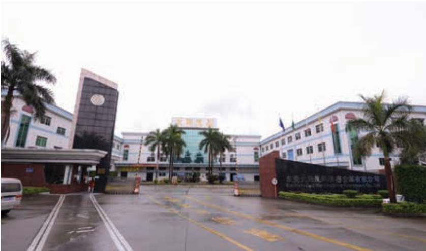
Sun Mansfield Plant
