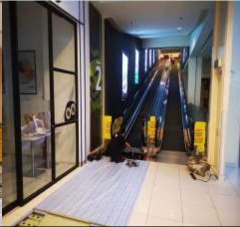
Replacement of traveller step chain and handrail
