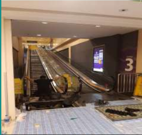
Replacement of traveller step chain and handrail
