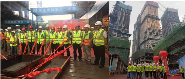
Topping Out Of Tower 3 (South)
