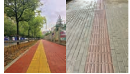
Wuxin permeable bricks used in sponge city projects in Wuhan
