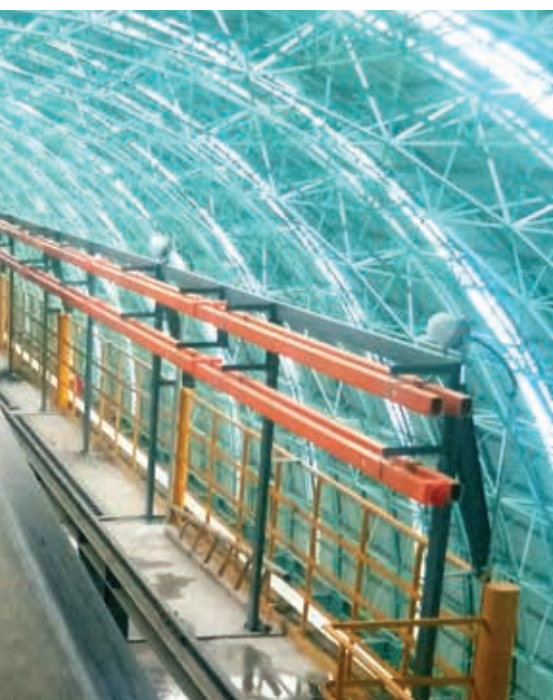
Photo: Slag transport to vertical roller mill by conveyor belt
