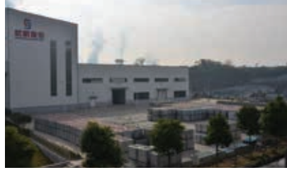
Key equipment is supplied by Hess Group GmbH
