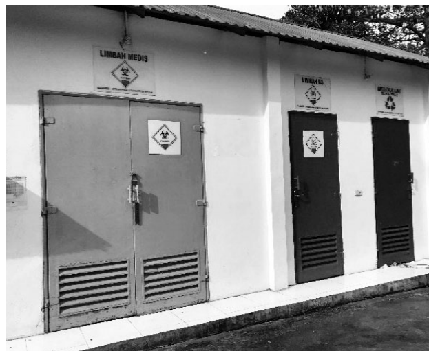
Designated rooms to isolate the sorted waste at Siloam Hospitals Lippo Village
