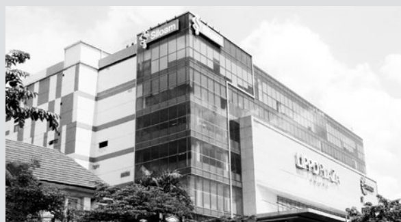
External View of SHYG
