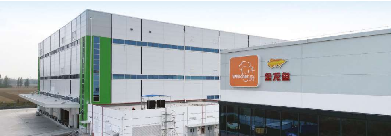
YKA employs specialised boilers to burn rice husks for energy as part of the circular economy of rice production in China.
