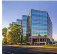
Haverty Furniture Co. Centrum at Glenridge / Central Perimeter 49,000 sf renewal
