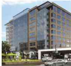
Crown Castle 8000 Avalon / North Fulton 55,600 sf new
