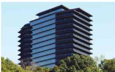
Three Ravinia / Central Perimeter $210M ($258 psf) Preferred Apartment Communities
