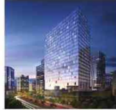
CBRE Three Alliance / Buckhead 105,000 sf new
