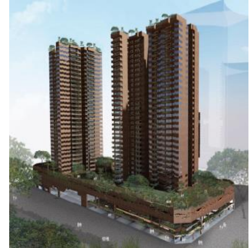
Tan Quee Lan Street Client: MTG Apartments Pte Ltd & MTG Retail Pte Ltd Approx Contract Value: S$227.5 million
