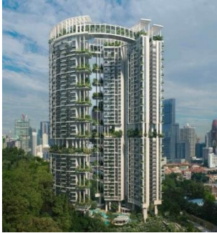
Pearl Bank Client: ARECA Investment Pte Ltd Approx Contract Value: S$190.0 million
