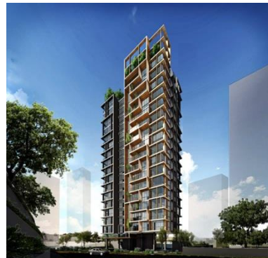
Cairnhill Rise Client: TSky Cairnhill (Private) Limited Approx Contract Value: S$24.3 million
