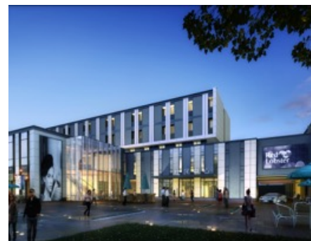
Riverbay Gardens, Community Center, Suzhou 江湾雅园，仁恒里，苏州
