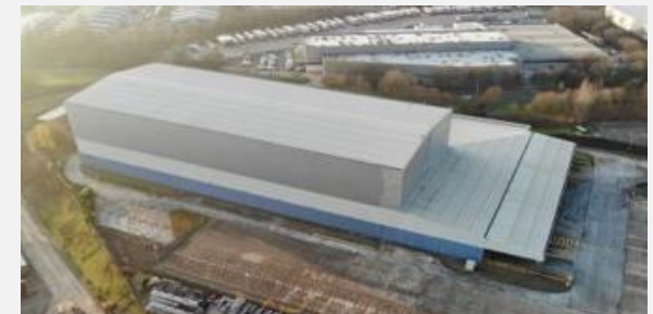
The Cube, United Kingdom Light industrial / logistics
