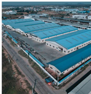
Apparel manufacturing facility, Callisto Apparel Co., Ltd (“ CA ”), Phnom Penh, Cambodia
