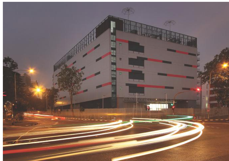
DataCentre One completed construction of 1-Net North and handed over the premises to the client.
