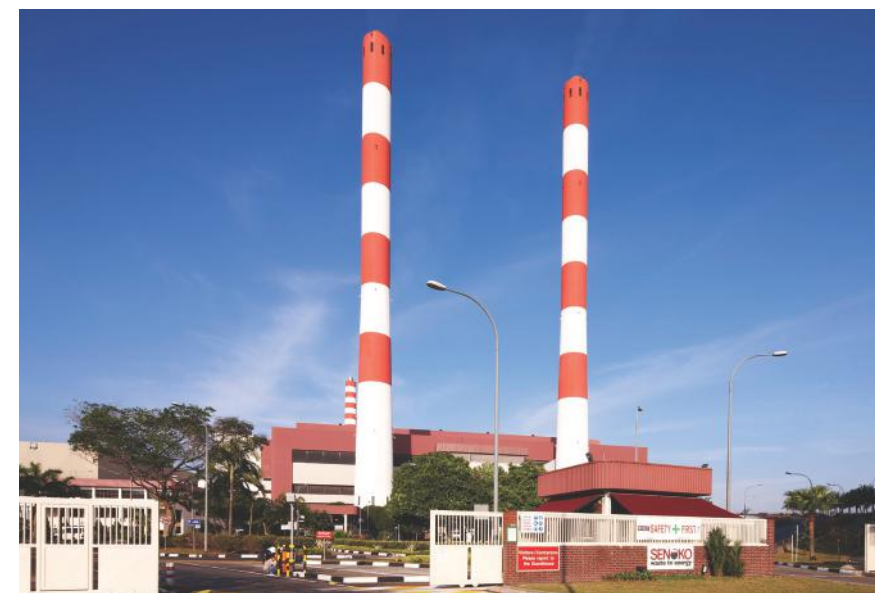
With the Senoko WTE Plant's contracted incineration capacity raised by 10% to 2,310 tonnes per day, the capacity payment from NEA has been correspondingly increased.
