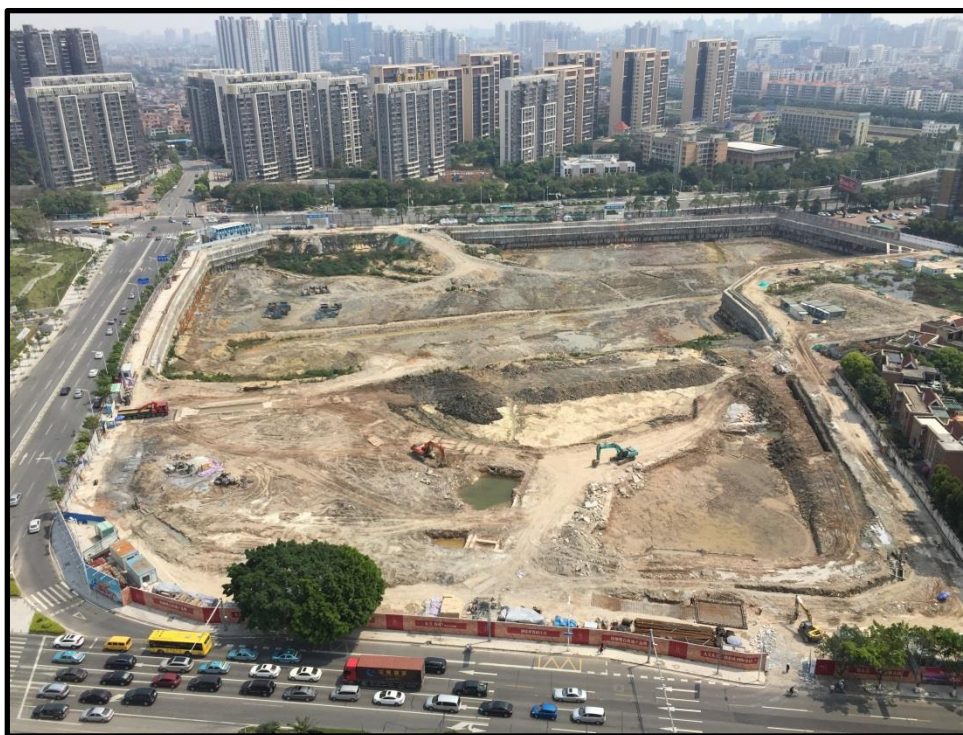
Site preparation works
