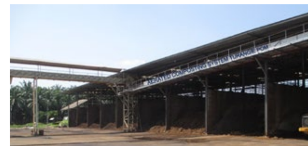
Aerated Bunker Composting at Turangie Palm Oil Mill, North Sumatra.
