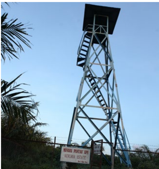
Fire Monitoring Tower at Kencana Estate, Rokan Hilir, Riau.
