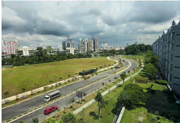
The clearing of the forest paved the way for the new Chuan Grove road; photo taken in April 2024
