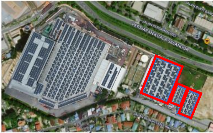
Shah Alam – Main Parking, CDE Warehouse & CDEW Parking (1,542 kWp)
