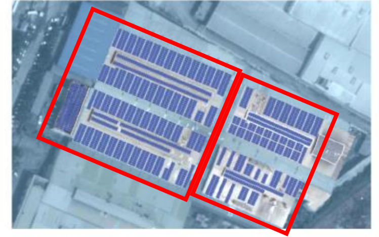
Lot 10, Rawang - 1,165 kWp
