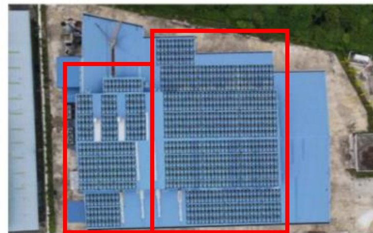
Lot 28, Rawang – 553 kWp
