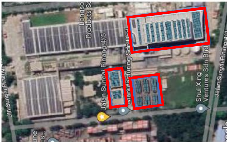
FNDM Pulau Indah (1,488 kWp) – Warehouse, Admin Block, Carpark Roof
