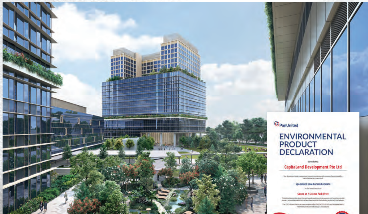
The Geneo, developed by CapitaLand, received the Environmental Product Declaration (EPD) for its use of specialised low-carbon concrete which helps to reduce embodied carbon. Artist's impression courtesy of CapitaLand.
