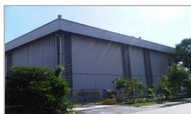
3 Kim Heng Warehouse 4 Penjuru Lane
